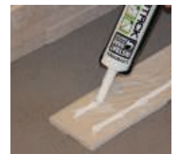
Applying Ritetack in stripes on tiles.
