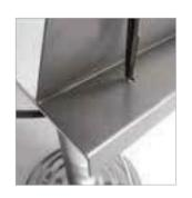
Lie the steel base over the board and mark the hole positions on the substrate
